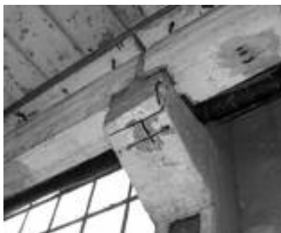
Fot. 1. Oparcie belek podsuwnicowych na skraju wspornika Photo 1. Crane girders support on the very edge of cantilever
