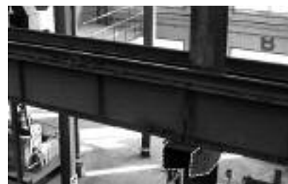
Fot. 1. Fragment podtorza suwnicy w obrębie słupa Photo 1. Part of the runway structure by the column
