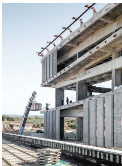
Photo 3. Assembly of the prefabricated concrete facade panels
