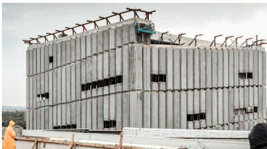
Photo 4. Prefabricated concrete panels used as finishing material of the facade
