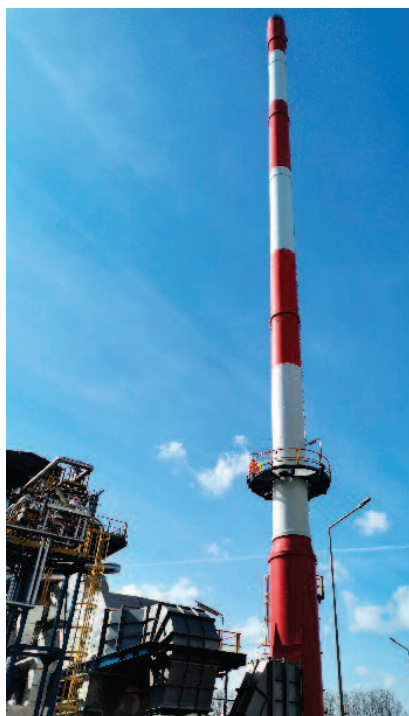
Photo 1. Self-supporting steel chimney with a height of 80 m [1]
