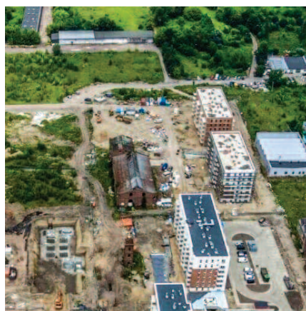
Photo 1. Construction of boiler and turbine plants in 2019 [12]
