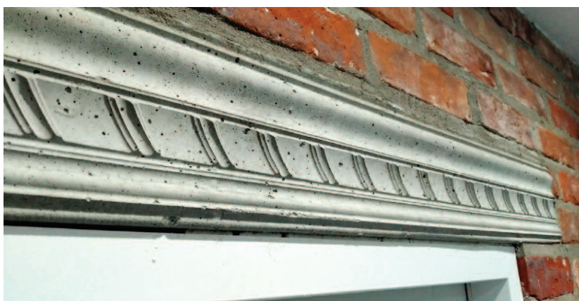
Photo 4. Fiber reinforced concrete lintel with a decorative face
