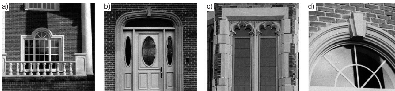
Photo 2. Decorative: a) window portals [11]; b) door portals [12]; c) lintels [13]; d) keystones [11]
