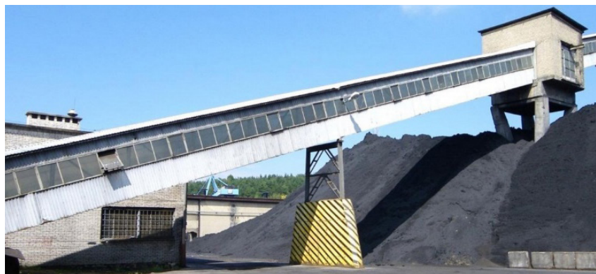
Photo 1. View of the oblique bridge
