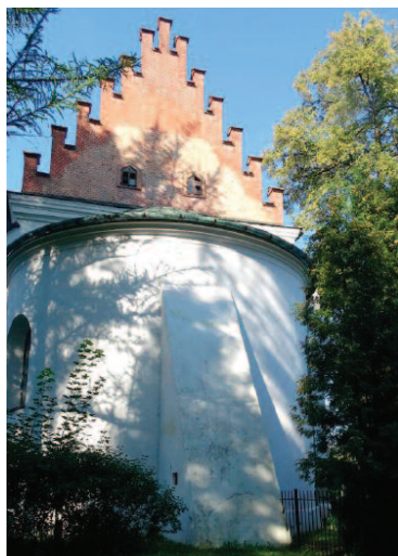
Photo 4. View of the buttress closing the apse
